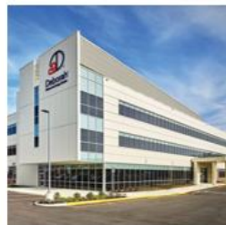
Medical Office Building, Browns Mills, NJ
